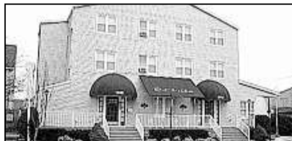
VIEW OF THE SEA MOTEL – SEASIDE HEIGHTS, NJ – FULL APPROVAL FOR 9 LUXURY CONDOS – U/C
