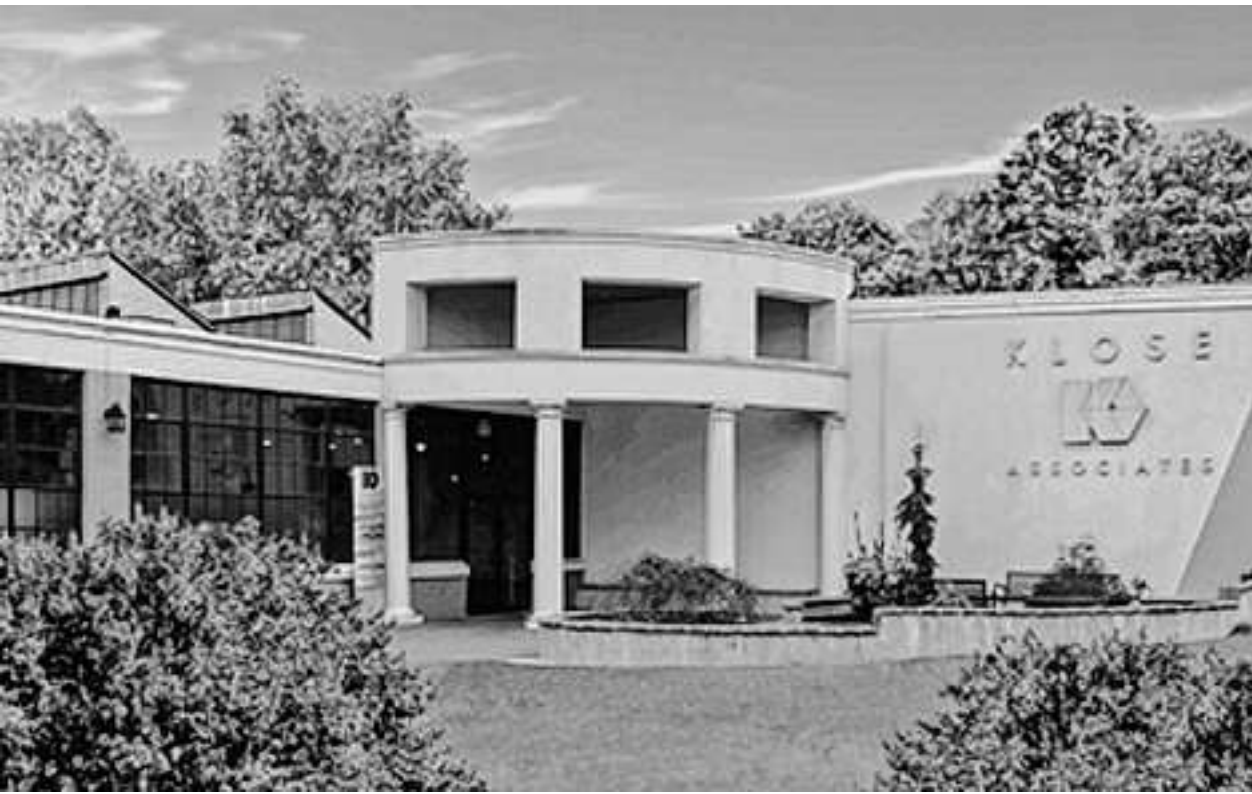
The "Factory At Broadway," located at 804 Broadway in West Long Branch. COURTESY OF WEICHERT REALTORS
